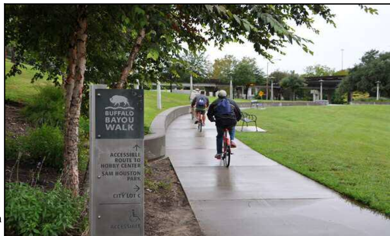
Figure 21.21 – Buffalo Bayou Trail – Caption: Everything in this photo below the highway bridges is designed to be flooded. This includes the lampposts lining the trail. They utilize two bulbs. If one bulb burns out, maintenance knows it is time to replace the bulb, but maintenance is not in a hurry to do so, because there is still light. Also, the park bench is bolted to a concrete base to prevent it from being washed away during high waters. – Source: author – [file:\BBT1071.jpg]
