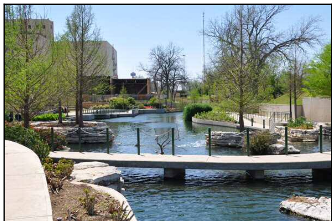
Figure 21.15 – New River Walk Section – Caption: This section is below the flood tunnel intakes at East Josephine Street. Notice how the river landscaping is more expansive than the downtown section and how it is integrated with its surrounding community. – Source: author – [file:\SA331.jpg]
