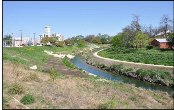
Figure 21.16 – Open Space Section on River Walk – Caption: This stretch is between the downtown section and the outflow of the flood control tunnel beneath the city. Although it looks like levees bordering the side of the river, it is really a channelized river bank in its normal banks. Note the manhole cover of the sanitation sewer system on the left side of the picture. – Source: author – [file:\SA304.jpg]
