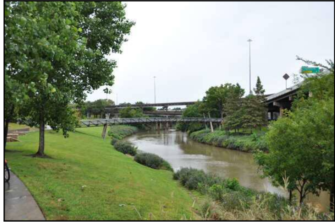
Figure 21.22 – Buffalo Bayou Trail – Caption: Everything in this picture except the highway bridges are designed to be periodically inundated. This includes the trail in the far left of the photo, the bridge across the bayou, and the vegetation lining the river. Native species tolerant to being inundated were planted on the river banks. – Source: author – [file:\BBT1059.jpg]
