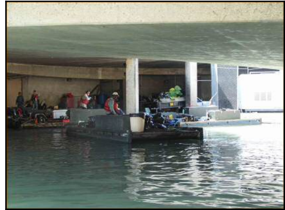
Figure 21.20 – Maintenance on the River Walk – Caption: A maintenance barge in the maintenance facility next to Gate #5 beneath East Nueva Street. – Source: author – [file:\RiverWalkMaintenance.jpg]
