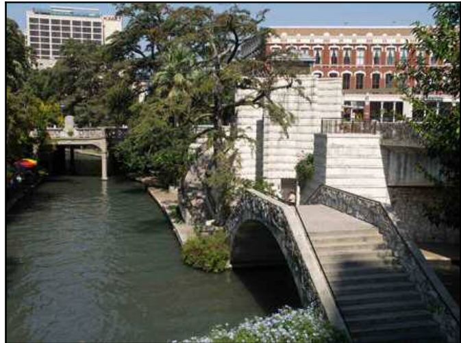
Figure 21.14 – Original Section of the River Walk – Caption: This scene is located at the junction of the branch to the Convention Center. Located below street level, it creates a quaint world of its own with little integration with the downtown community surrounding it. – Source: author – [file:\pwrpt018riverjunction.jpg]
