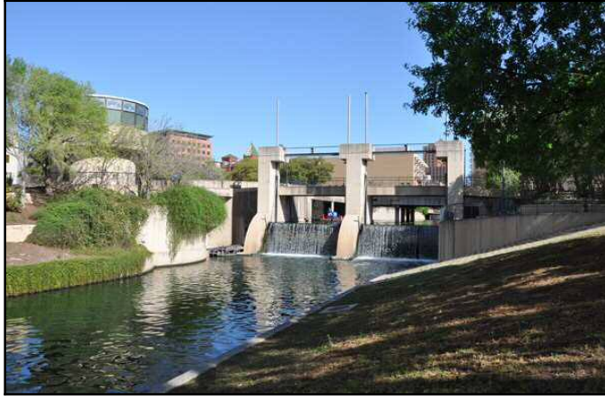
Figure 21.19 – Gate #5 beneath East Nueva Street – Caption: The maintenance area in figure 21.18 is located to the left of the dam. The gates can be raised in times of flood, or the gates can be raised and the downtown section drained to allow heavy equipment access to the area. The riverbed becomes the access road for maintenance. – Source: author – [file:\SA345.jpg]
