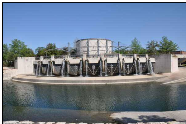
Figure 21.18 – Out-take of San Antonio Flood Control Tunnel – Caption: The out-take of the tunnel underneath San Antonio. – Source: author – [file:\SA295.jpg]
