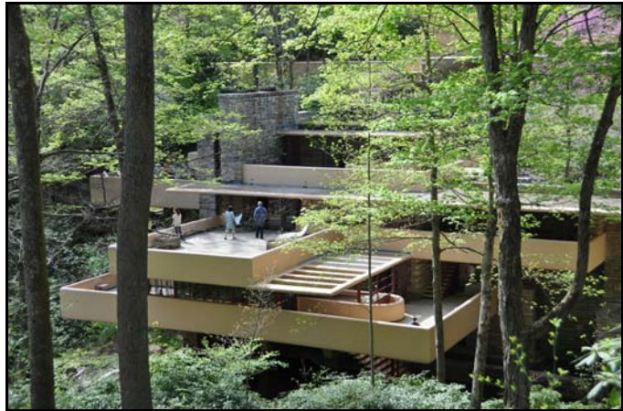
Figure 16.38: Sunshading – Looking west, this is a view of Fallingwaters depicts the impacts of the sun and the concept of sunshading. During the summer, the deciduous trees help to provide protection from excessive solar heating. During the winter, it encourages heating and the balconies become heat sinks that radiate stored solar radiation. Source: Author – [file:\FW154.jpg]
