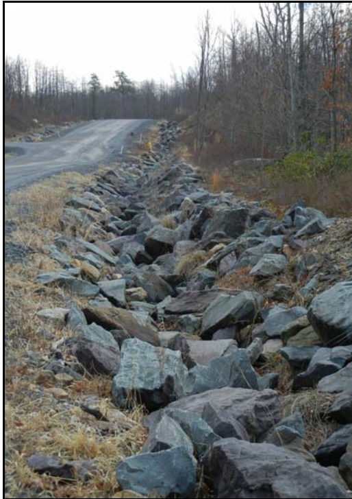
Figure 16.27: Infiltration Trenches – Filling raceways with rock aggregate slows the speed of the water and encourages greater water infiltration. – Eagle Rock, near Hazelton, PA. Source: Source: author – [file:\ER1254.JPG]
