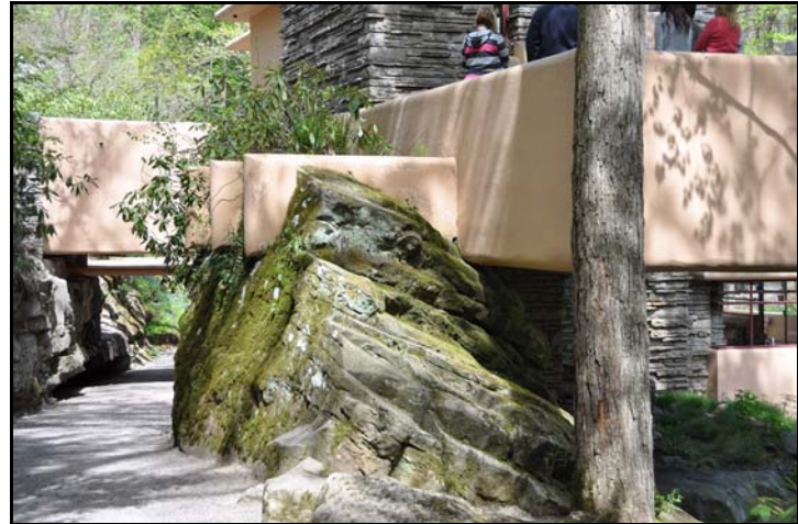
Figure 16.36: Connective Concrete Beams – Illustrating the aesthetic design with nature is the use of three concrete beams to link the house with the rock outcropping. They serve no functional purpose. Fallingwaters, Ohio, Pennsylvania. Source: Author – [file:\FW130.jpg]
