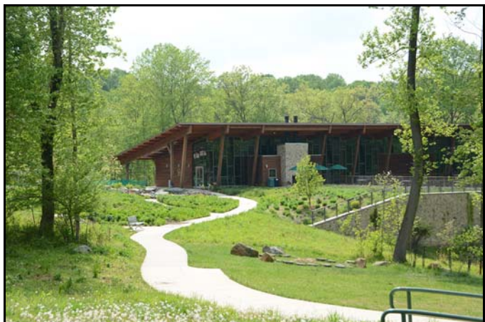
Figure 16.39: Robinson Nature Center – The Robinson Nature Center is a demonstration facility for LEED and sustainability by Howard County and Maryland Department of Natural Resources. As a footnote, the green roof in Figure 16.18 is visible in this photo between the stone wall and main building. Howard County, Maryland. Source: author – [file:\RNC001.jpg]
