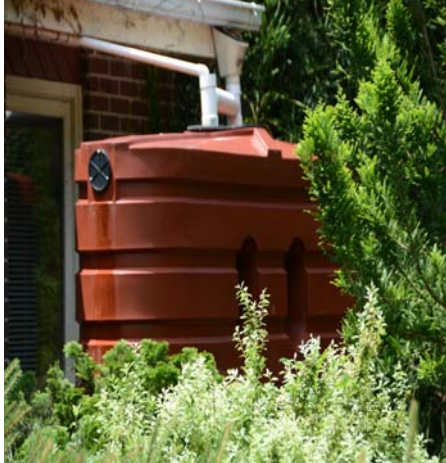
Figure 16.21: Above Ground Cistern – Rainwater can be collected and stored in a holding tank or cistern where it can be used for irrigation, ponds or wetlands, or released at a later date to infiltrate the ground. This above the ground cistern collects rainwater and can use a gravity feed to water plants at a later date. Note the small pipe is from the air conditioner. Brookside Gardens, Wheaton, Maryland. Source: author – [file:\BSG-020[gd].JPG]
