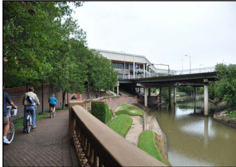
Figure 16.30 – Buffalo Bayou Trail – Caption: Everything in this picture including the trail on the left are designed to be periodically inundated with flood waters. Good design can facilitate healthy waterways along with park and recreation uses. – Source: author – [file:\BBT1058.JPG]
