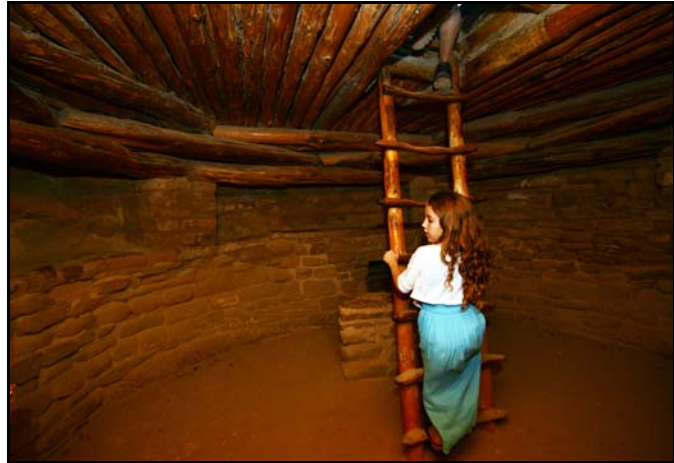
Figure 16.11: Hot Arid: Kiva – Kiva construction is an underground dwelling construction. The walls are hollowed out of the ground and the roof is lined with juniper logs and covered over with dirt. The structure will moderate temperatures. Mesa Verde National Park, Colorado. Source: author – [fig:\MV166[vg].jpg]
