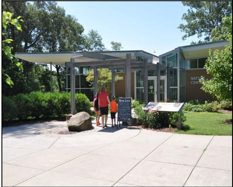
Figure 16.22: Below Ground Cistern – Aesthetically pleasing and functional, the nature center’s two roofs funnel rain water into the channel above the walkway which drains with a waterfall into the cistern underneath the large rock. Killens Pond State Park Nature Center, Felton, Delaware. Source: author – [file:\KP002[gd].jpg]
