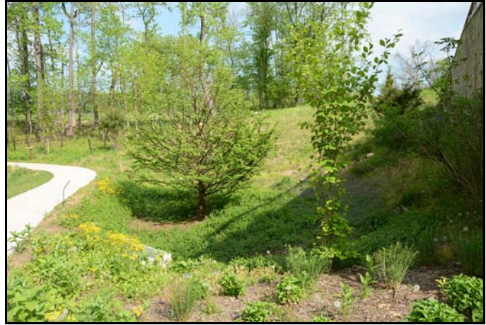
Figure 16.25: Rain Gardens/Rain Pockets – Rain gardens are small depressed areas that can capture and temporarily hold water until it is absorbed into the ground or absorbed by the plants. Robinson Nature Center, Howard County, Maryland. Source: author – [file:\RNC024.JPG]
