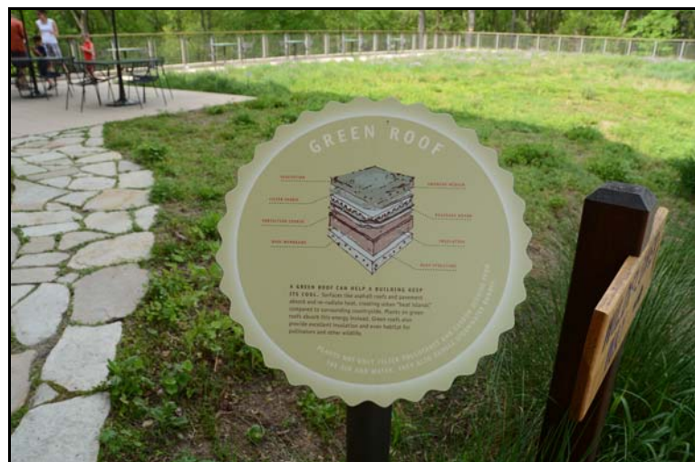
Figure 16.18: Robinson Nature Center Green Roof – Normal roofs collect and quickly disperse the water through down spouts away from the building. Green roofs are the first line of stormwater management. They hold water and slow its dispersal. It returns the system to a more natural state. Robinson Nature Center, Montgomery County, Maryland. Source: author – [file:\RNC005.jpg]
