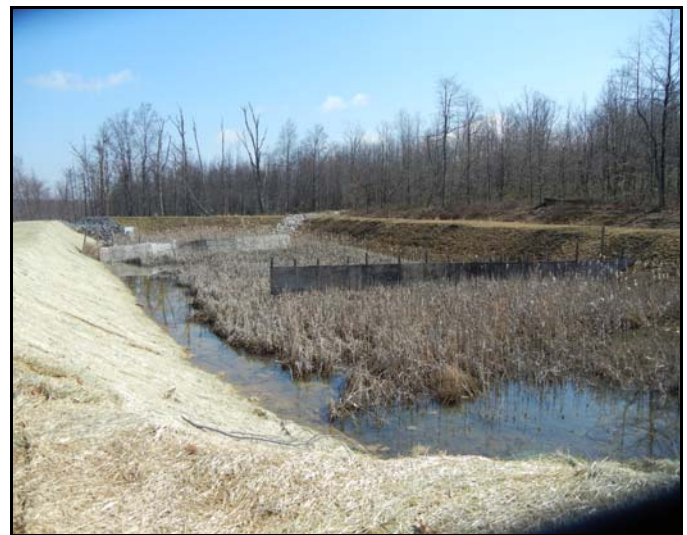
Figure 16.26: Retention Areas – Conceived in the 1990s, retention areas have become the most widely used storm water management technique. Water enters from the lower right corner of the photo where the retention area with natural vegetation holds the water. A second entry point is in the upper right corner of the photo. The out-take is in the upper left corner of the photo. Eagle Rock, near Hazleton, Pennsylvania. Source: author – [file:\ER1239.jpg]
