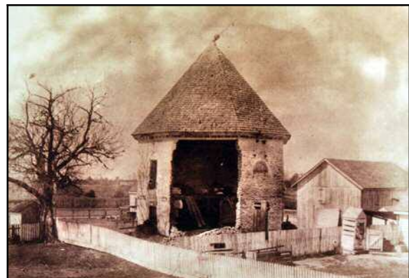
Figure 14.7 – Magazine (before restoration) – Caption: The Magazine before restoration. A portion of the wall of the Magazine is missing as is the wall surrounding the Magazine. – An original sketch of the Magazine at Williamsburg provides a good guide in the restoration of the building. – Source: Yetter, G., (1988) [file:\fig1305-WB106.jpg]
