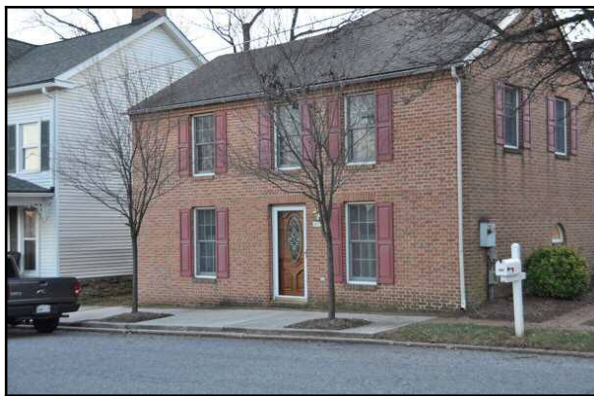
Figure 14.23 – House in Burkittsville (front) – Caption: Located in a historic district, the front of the homes conforms to height, proportion, and setback rules. Also, note that the brickwork is a Flemish Bond. – Source: Author [file:\fig1323-Burkittsville016.JPG]
