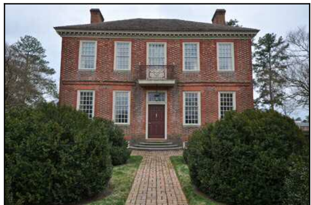
Figure 14.4 – Lightfoot House – Caption: The Lightfoot House is an example of a building that for the most part needs preservation. – Source: author [file:\fig1304-WB037.JPG]
