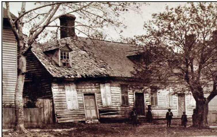
Figure 14.12 – John Crump House (before) – Caption: In Williamsburg, the John Crump House was razed in 1893. Since it is located on the Duke of Gloucester Street along with other establishments, it was important to reconstruct the house to be consistent with other buildings. It was reconstructed in 1941 (figure 14.11). The original photo provided important source material for the reconstruction. Note that a tree was planted where there was originally a tree in the photo – Source: Yetter, G., (1988) [file:\fig1310-WB109.jpg]
