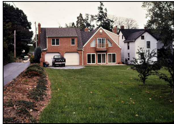
Figure 14.24 – House in Burkittsville (rear) – Caption: The rear of the same house in Burkittsville. People are allowed non-conforming designs. It is a compromise between maintaining historical integrity and modern designs and convenience. – Source: author [file:\fig1324-Burkittsville003.JPG]
