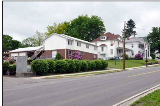
Figure 14.22 – Frostburg Ambulance – Caption: Located in a historic district, it shows improper setback, proportion and a facade that is inconsistent with the surrounding buildings. Frostburg, Maryland. – Source: Author [file:\fig1322-HP25ambulance.jpg]
