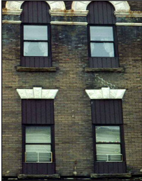
Figure 14.33 – Windows – Caption: At one time this building had majestic windows. Close inspection reveals three indicators: The new brickwork (Note the difference in mortar colors), the large arched lintels embedded in the brick wall, and the original sills. – Source: author [file:\fig1333-BlockDown[3].jpg]
