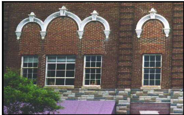
Figure 14.33 – Windows – Caption: At one time this building had majestic windows. Close inspection reveals three indicators: The new brickwork (Note the difference in mortar colors), the large arched lintels embedded in the brick wall, and the original sills. – Source: author [file:\fig1333-BlockDown[3].jpg]
