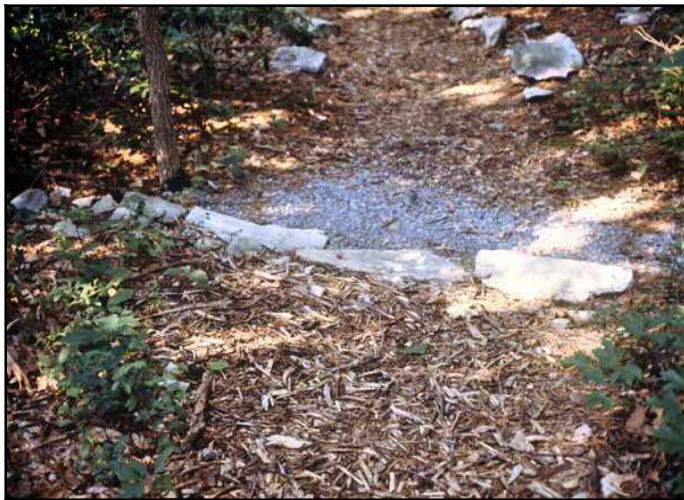
Figure 13.31: Waterbar (stone) – An example of a stone waterbar. Note that it utilizes only one row of rocks and an attempt was made to interlock the rocks. The view is looking uphill and the water is diverted to the right in the picture. Gambrill State Park, Maryland. Source: Author – [file:\DSC_0149.jpg]
