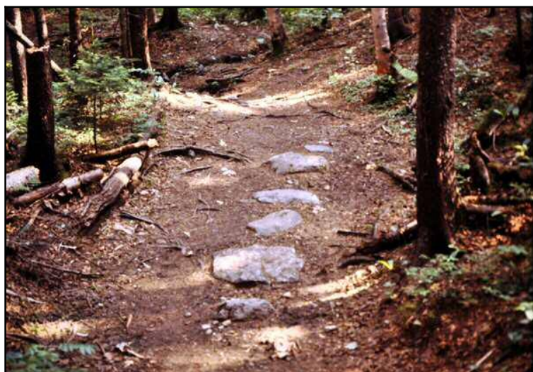
Figure 13.45: Ineffective Stone Walkway – This section of the trail demonstrates the improper use of stepping stones on the trail. Most hikers will simply hike on the compacted trail to the left of the rocks and avoid the even slight unevenness of the stepping stones. White Mountains, New Hampshire. Source: Author – [file:\T1410-ImproperSteppingStones.JPG]
