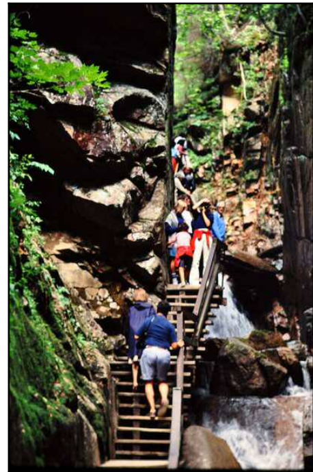
Figure 13.12: Planked Tread – The typical plank tread steps are illustrated at the Flume in Franconia Notch. Flume, Franconia Notch, New Hampshire. Source: Author – [file:\fig1255-T317.JPG]
