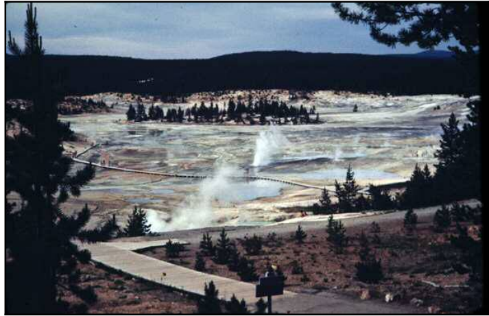
Figure 13.49: Yellowstone Boardwalk – This is a low level boardwalk traversing the hot springs at Yellowstone National Park. Notice how the walkway harmonizes with the landscape. However, since there are no railings, some would raise a safety concern. Yellowstone National Park, Wyoming. Source: Author – [file:\T1017-DSC_0189.JPG]
