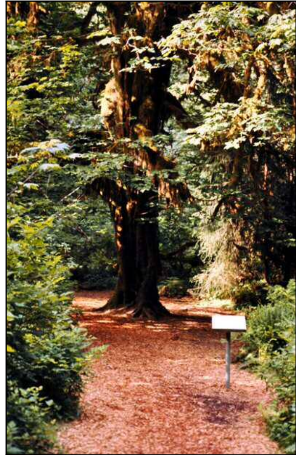
Figure 13.22: Olympic Trail – The wood chip trail surfacing provides a clear and obvious trail to follow, and it provides a quiet walkway consistent with the experience. Olympic National Park. Source: Author – [file:\OlympicTrail-S113.jpg] [alt file:\DSC_0139.JPG]
