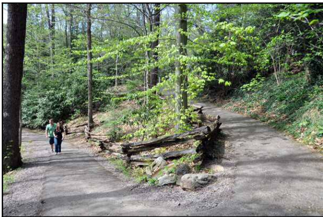
Figure 13.6: Switchback at Fallingwaters (View #1) – The switchback creates a gentler slope for the trail. This scene shows the trail switching back on itself to gain vertical elevation without having to use steps. Fallingwaters, Ohio, Pennsylvania. Source: Author – [file:\fw097switchback.jpg]
