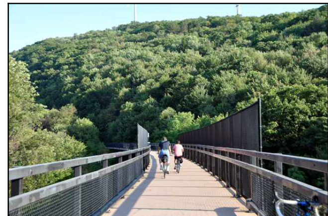
Figure 13.43: Viaduct – On the Great Allegheny Passage rails-to-trail, this viaduct crosses a railroad, automobile road, and stream. In doing so, this viaduct avoids three different conflicts. Near Myersdale, Pennsylvania. Source: Author – [file:\GAP029viaduct156.jpg]
