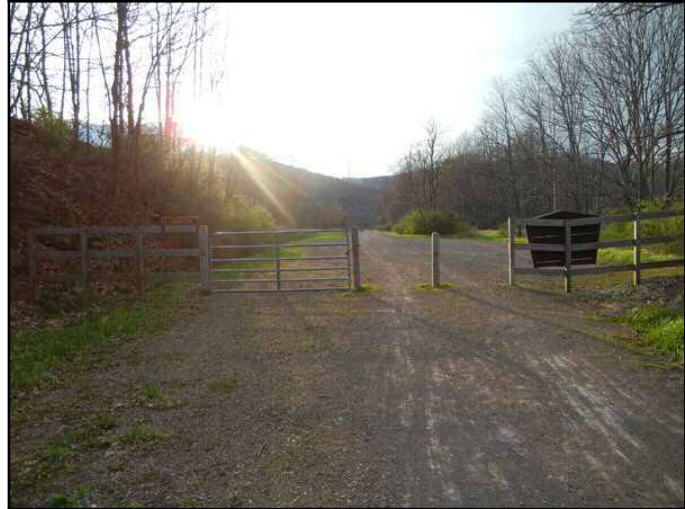
Figure 13.39: Sandpatch Gate and Bollard – To provide access, this area utilizes both a removable bollard and gate. Removing the bollard allows access of the rails-to-trail by emergency and maintenance vehicles. Sandpatch, Pennsylvania. Source: Author – [file:\GAP028sandpatch001.jpg]
