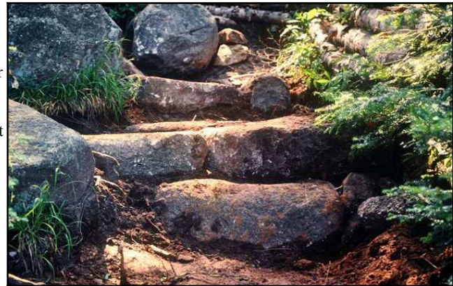
Figure 13.10: AMC Steps, Waterbars, and Brush – The AMC (Appalachian Mountain Club) recently completed this trail section. The brush piled on the right encourages the use of the steps and discourages use of the old trail (i.e. where the brush is piled). The waterbar below the steps diverts water off the trail. In two years, this site will look completely natural. Boot Spur, White Mountains. Source: Author – [file:\T905-RockSteps.JPG]
