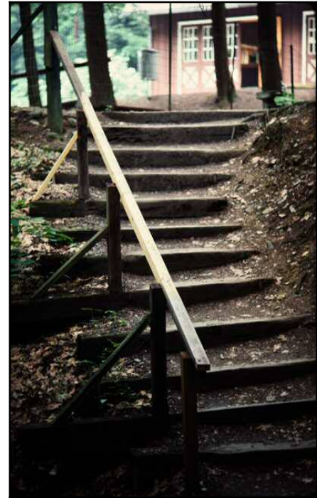
Figure 13.13: Log or Timber Raiser – A typical timber raiser steps where railroad ties are used to create the step. The area behind the step is backfilled up to the next step. – Dingman's Ferry, Pennsylvania. Source: Author – [file:\T312-RRsteps.JPG]
