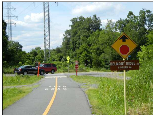
Figure 13.42: Auto Crossing – A bridge at this location would avoid conflict between bikers and automobiles. W&OD Trail, Ashburn, Virginia. Source: Author – [file:\W&OD008.jpg]
