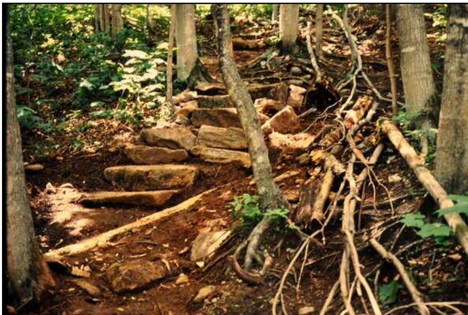
Figure 13.10: AMC Steps, Waterbars, and Brush – The AMC (Appalachian Mountain Club) recently completed this trail section. The brush piled on the right encourages the use of the steps and discourages use of the old trail (i.e. where the brush is piled). The waterbar below the steps diverts water off the trail. In two years, this site will look completely natural. Boot Spur, White Mountains. Source: Author – [file:\T905-RockSteps.JPG]
