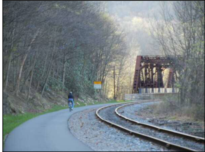
Figure 12.8: GAP Trail – The Greater Allegheny Passage Trail is a converted Western Maryland rails-to-trails. Marketed as a trail for through travelers, most of its use is by local citizens. Also, showing that different uses can share the same right-of-way, the trail shares the right-of-way along this stretch with a scenic steam railroad. Cumberland, Maryland. Source: author – [file:\GAP002trail002.jpg]
