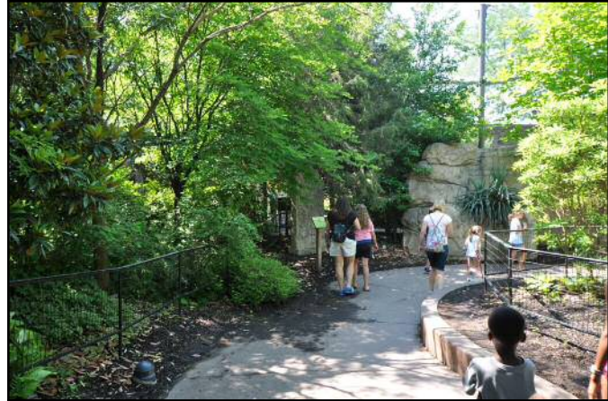
Figure 11.18: Mesh Fence – The black colored fence is fairly unobtrusive and easily blends into the background. Note the soil compaction on the right side between the curb and fence. The curb is sufficiently wide to encourage many children to use the curb as a balance beam to walk around the bend in the trail. Source: author [file:\PHZ0881.jpg]
