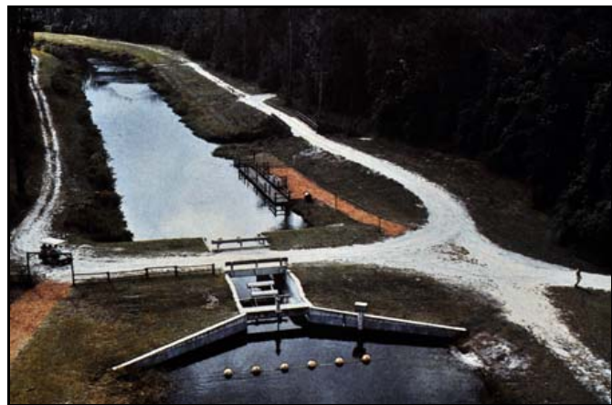
Figure 6.8 – Canals and Dams – Caption: Flood control is an important consideration. It is also an environmental concern. The objective is to drain flood waters, but maintain a high water table during normal periods. The water-control structures helps to accomplish this objective. Magic Kingdom, Disney World, Orlando, Florida. – Source: Author [file:\fig0608-DSC_0057.JPG]
