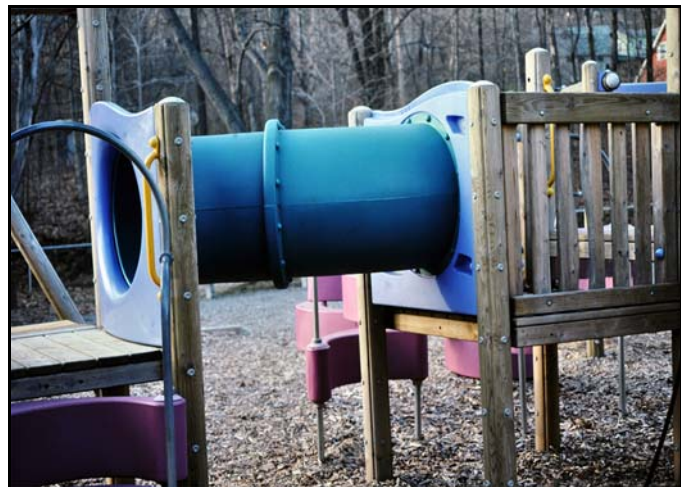
Figure 3.23: Barriers – On elevated platforms, barriers should be a minimum of 38" high and should not encourage climbing on them. Frostburg, MD. Source: author [file: \DSC_0061.jpg]
