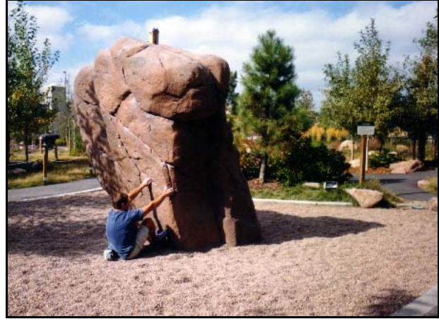
Figure 3.29: Bouldering Rock – The bouldering rock outside of REI demonstrates the application of the safety standards to non-playground play. The fall zone is adequate and the pea gravel is an appropriate surfacing. Denver, Colorado. Source: author [file: \rei07boulder.jpg]
