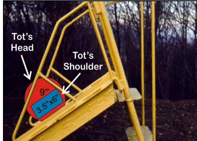
Figure 3.17: Head Entrapment – The head of tots (5-12) is bigger than their shoulders. A potential head entrapment exists if a 3.5"x6" rectangle (shoulders) can pass through an opening but a 9" circle (head) can't. Source: author [file: \PL_HeadEntrapment.jpg]
