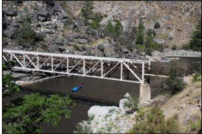
Figure 1.24: Frank Church Wilderness Bridge – A bridge across the Middle Fork of the Salmon in the Frank Church Wilderness Area. Although there are many reasons to build the bridge, is it really an appropriate structure in and experience for a Wilderness Area? Frank Church Wilderness, Idaho. Source: author – [file:\fig0119-DSC_0235.JPG]
